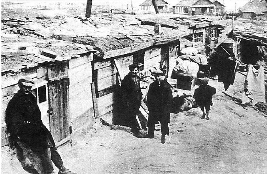
A photograph of workers' living accommodation at the Dnieper Dam site in 1931.
