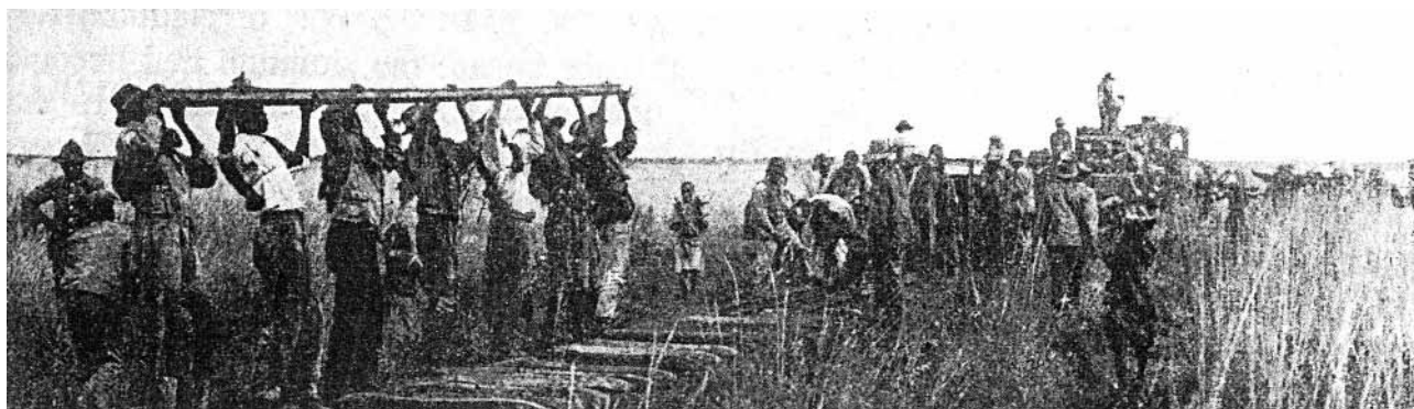
Construction of the Otavi Railway.
