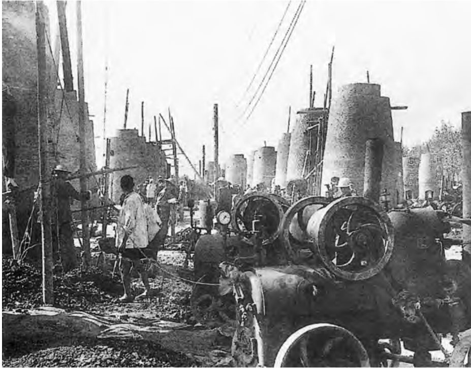
'Backyard' steel furnaces built during the Great Leap Forward.
