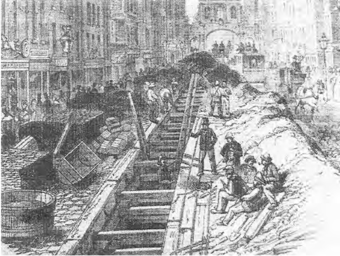
Building a sewer in London in 1844.
